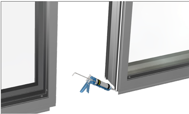
Fig 3. Apply sealant to the male snap feature, along its entire length, and then snapping the windows together.
